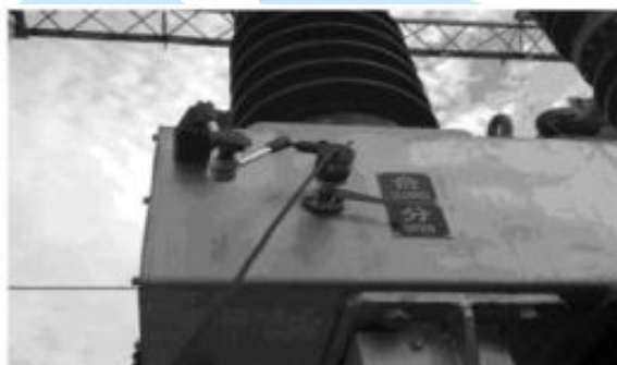
Installation of 35KV SF6 Switching Sensor
