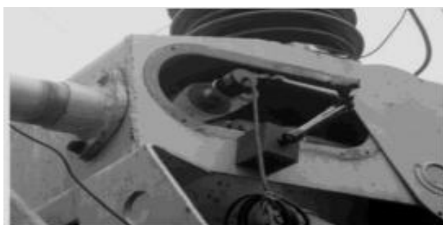
Installation of 110KV SF6 Switching Sensor
