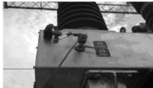
Installation of 35KV SF6 Switching Sensor
