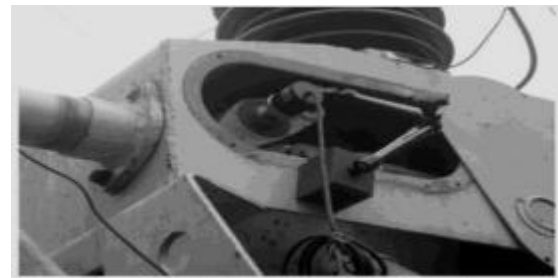
Installation of 110KV SF6 Switching Sensor
